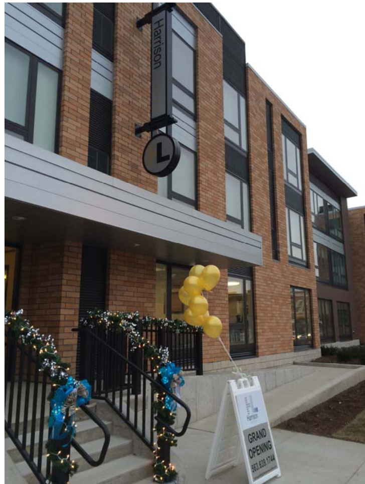
Harrison Lofts, an $11 Million infill redevelopment project funded in part with Neighborhood Stabilization Program Funds as well as Low Income Housing Tax Credits, opened in December 2013.
