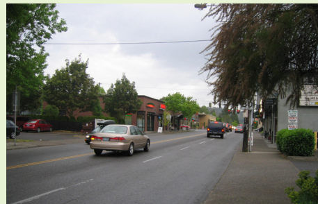
On an undivided four-lane road, cars waiting to turn left can block the travel lane, creating delays during peak travel periods and causing following drivers to change lanes as they go around turning cars
