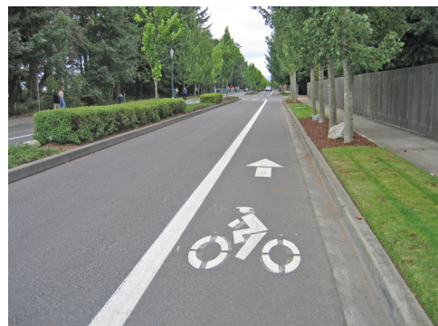
Bicycle lanes are the preferred bicycle facility if sufficient roadway space exists
