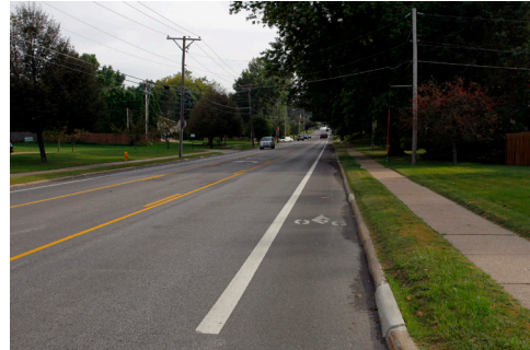
Transportation options: existing on-street bicycle lanes on Jersey Ridge Road.
