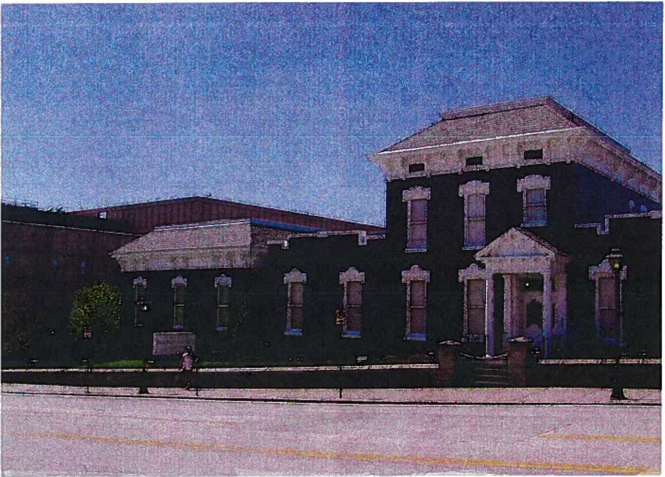
Above: The Halligan-McCabe Devries Funeral Home, 614 Main Street, Davenport, Iowa provides a good example of an addition that closely replicates the original historic architecture of a building. The average person would likely have a difficult time telling that the portion of the building to the left is a modern addition.
