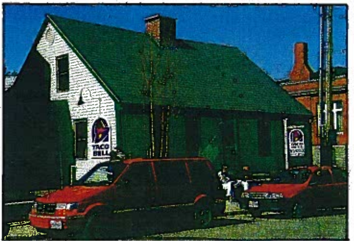
Taco Bell, Freeport, Maine. Most of the town's chain stores and franchises are in existing historic buildings.
