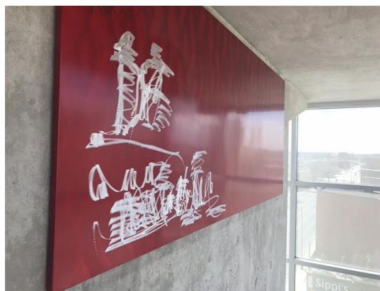
Graffiti on the wall of the Redstone Ramp
