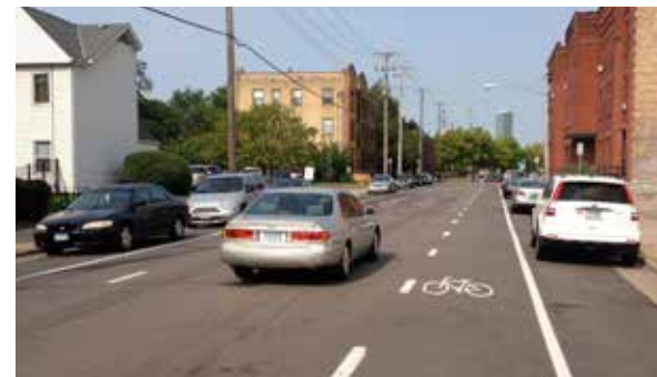
Bike lane symbols and lane stripping tell motorists and cyclists where to position themselves.
