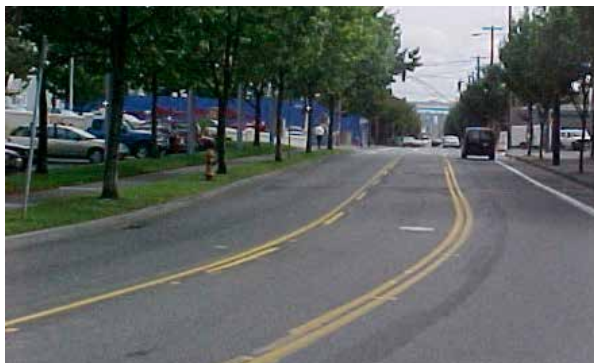
A climbing lane is added on the uphill portion of the roadway.
