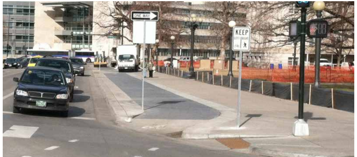
Raised separated bikeways are bicycle facilities that are vertically separated from motor vehicle traffic.
