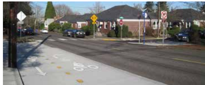
Separated Bike Lane Connection
