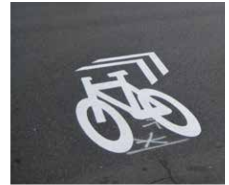
Some cities use pavement markings to indicate required turns or jogs along the bicycle route.
