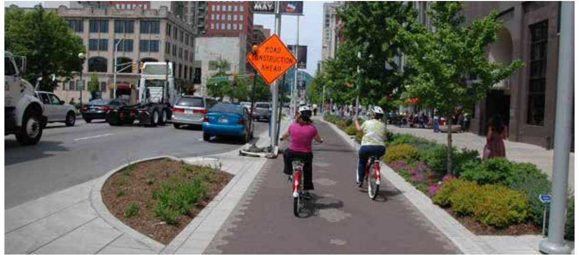
Raised separated bikeways are bicycle facilities that are vertically separated from motor vehicle traffic.
