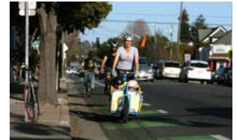
A colored bicycle lane on Laurel Street in Santa Cruz, CA alerts users to potential merging in advance of an intersection. Photo by Richard Masoner via Flickr (CC BY-SA 2.0).
