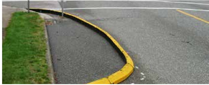
Temporary Curb Extension
