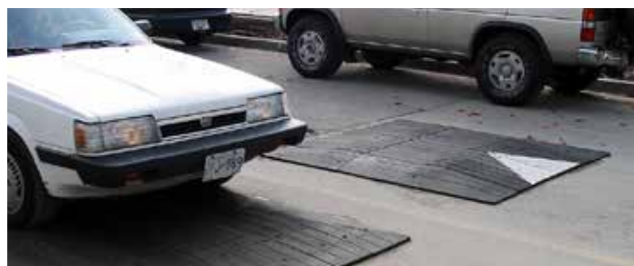
Temporary Speed Cushion
