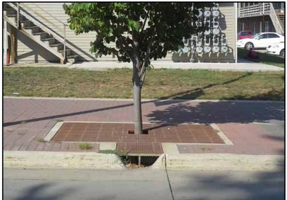
Figure 8. Tree well with Stormwater Inlet and Tree Grate
