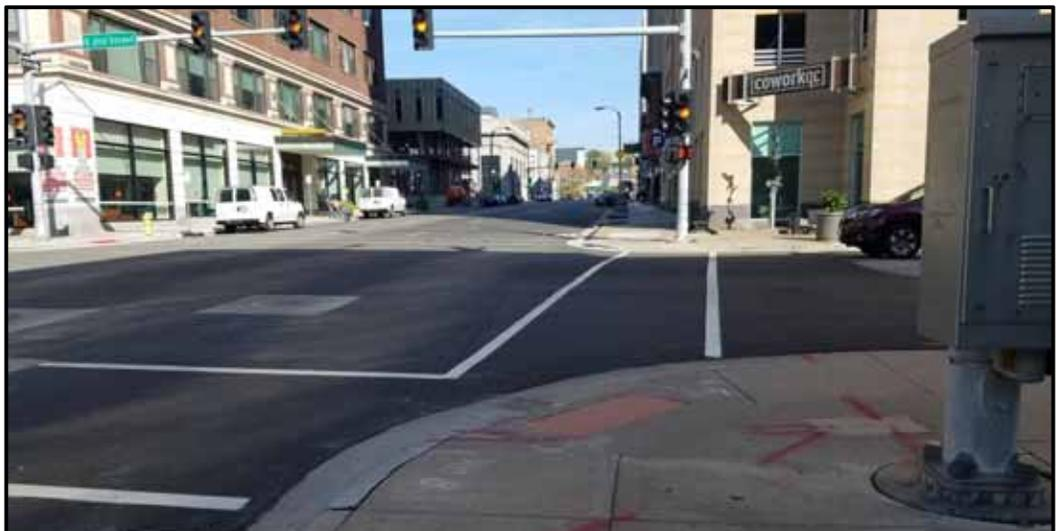
**Figure 14. Misaligned Crosswalk due to Corner Ramp.**
